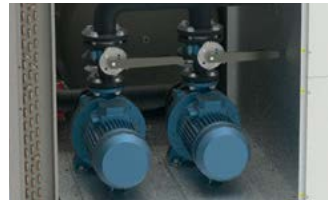
Pump section with or without storage tank.
